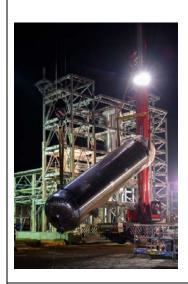
The reaction vessels for the new hydrogenation plant at Haltermann Carless' site in Speyer, Germany, are 9m long with a diameter of 2m and weigh 18 tons.
