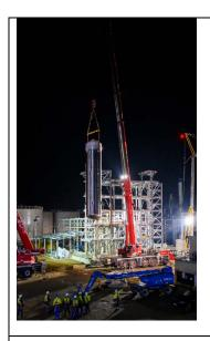
The reaction vessels for the new hydrogenation plant at Haltermann Carless' site in Speyer, Germany, are 9m long with a diameter of 2m and weigh 18 tons.
