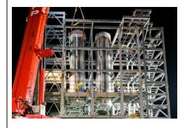
The reaction vessels for the new hydrogenation plant at Haltermann Carless' site in Speyer, Germany, are 9m long with a diameter of 2m and weigh 18 tons.
